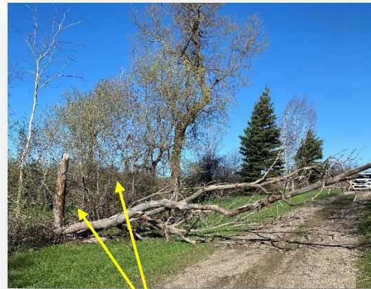
Lines still energized even with tree pulling them down (retrieved from Lake Region's Facebook)
